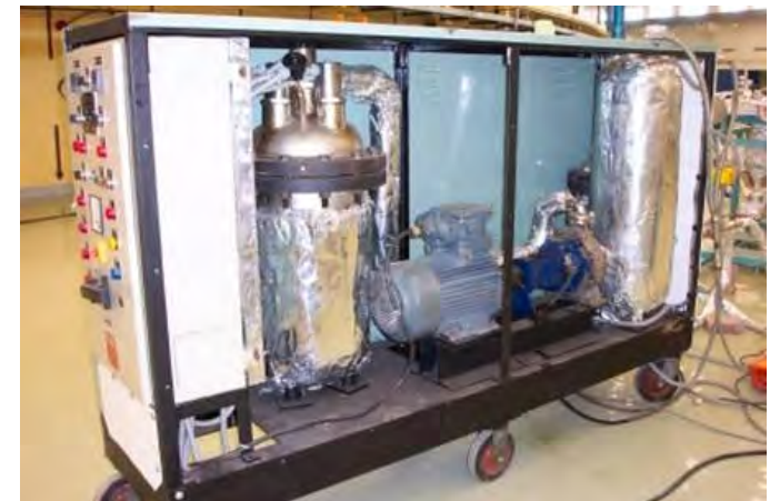
Super Heated Water Generator
